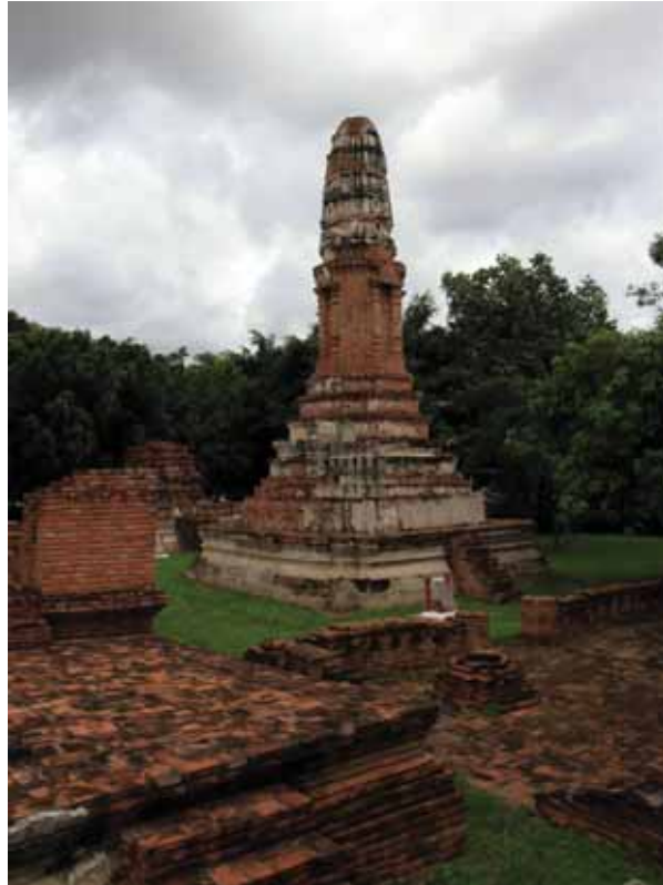
Illustration 2. The ruin of Wat Borom Phuttharam, The north-facing temple built during the reign of King Phetracha (ca. 1688 – 1703).
